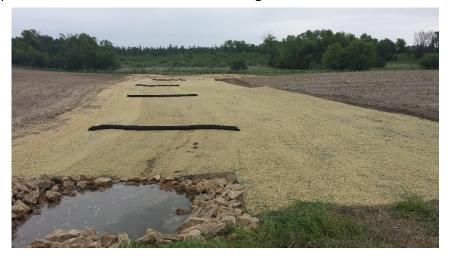
On a second field, a gully had formed as water flowed through the agricultural field. In this case, a water and sediment control basin was installed to temporarily hold back water. A perforated outlet pipe allows the water to slowly drain to a protected outlet location.
