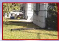
A very simple step you can take to reduce runoff from your yard is to redirect downspouts so that they empty into the yard where the water has a chance to infiltrate. Do not direct downspouts onto a side walk or driveway
