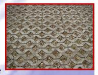
gaps between the pavers that allow water to soak through. The gaps can be filled with gravel or even seeded to allow small plants to grow. They are great for driveways, sidewalks or patios.
